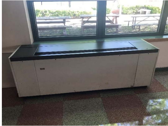
Typical Unit Ventilator
